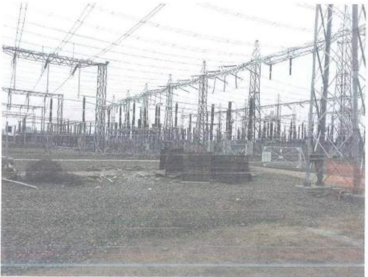
CIVIL AND ERECTION WORKS AT THE 220KV DANDORA SUBSTATION
